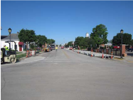
MAIN AT GRAND LOOKING WEST — BEFORE
