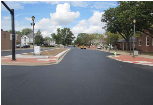
STREETSCAPE ON MAIN AT CENTRAL AVE—NORTH
