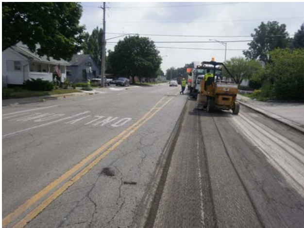
DAYTON DRIVE DURING CONSTRUCTION
