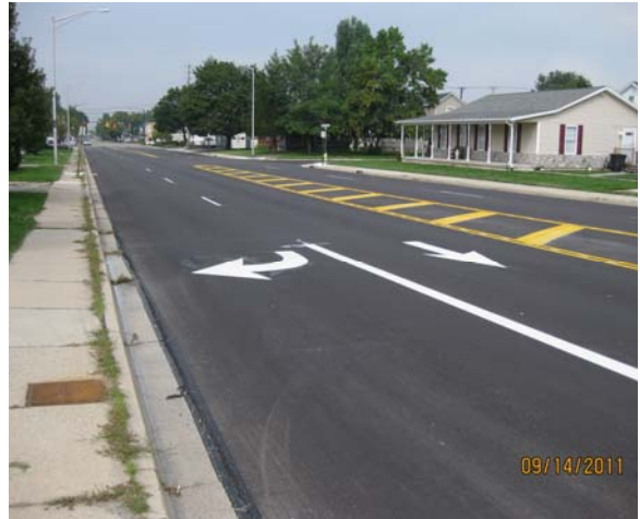
DAYTON DRIVE AFTER IMPROVEMENTS
