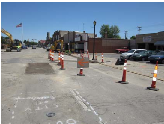
MAIN AT GRAND LOOKING EAST — BEFORE
